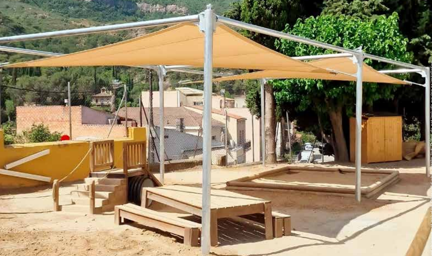
Installation of self-supporting shade in Monistrol de Montserrat
